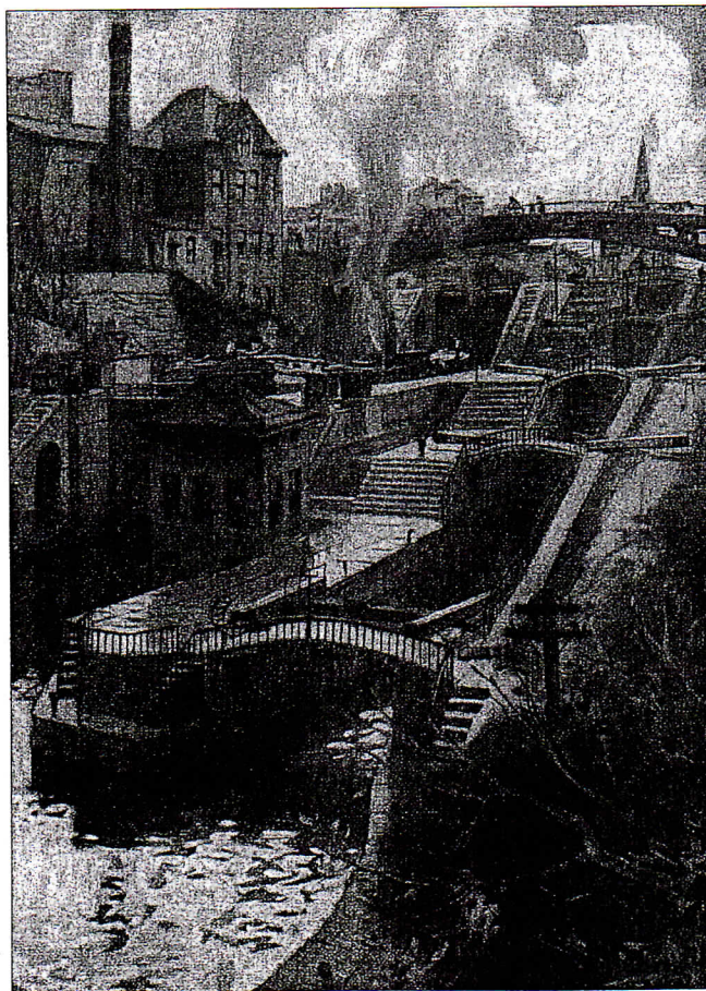
In Lockport, NY, canal boats climbed up and down a series of locks like a flight of stairs.
